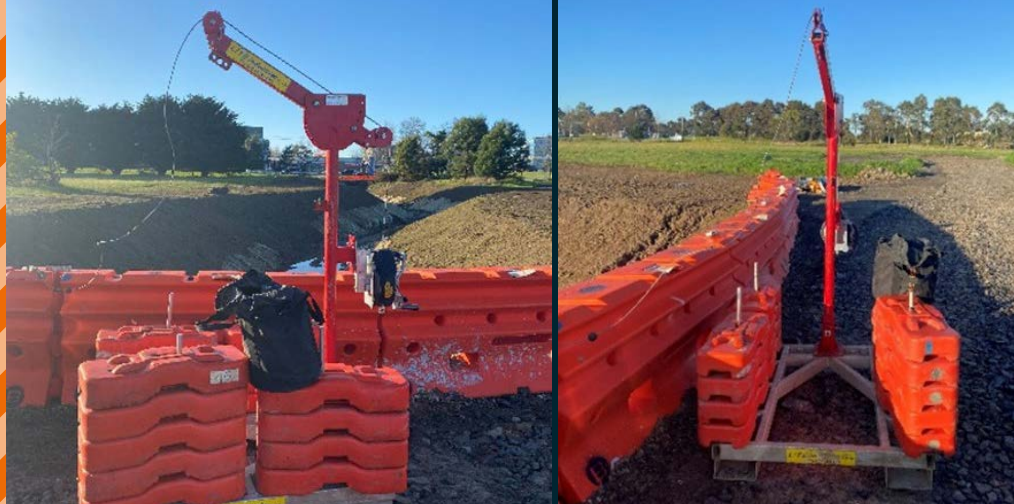
Mobile Davit Arm and trench view (left), using concrete temporary fence blocks as counterweight (right).
